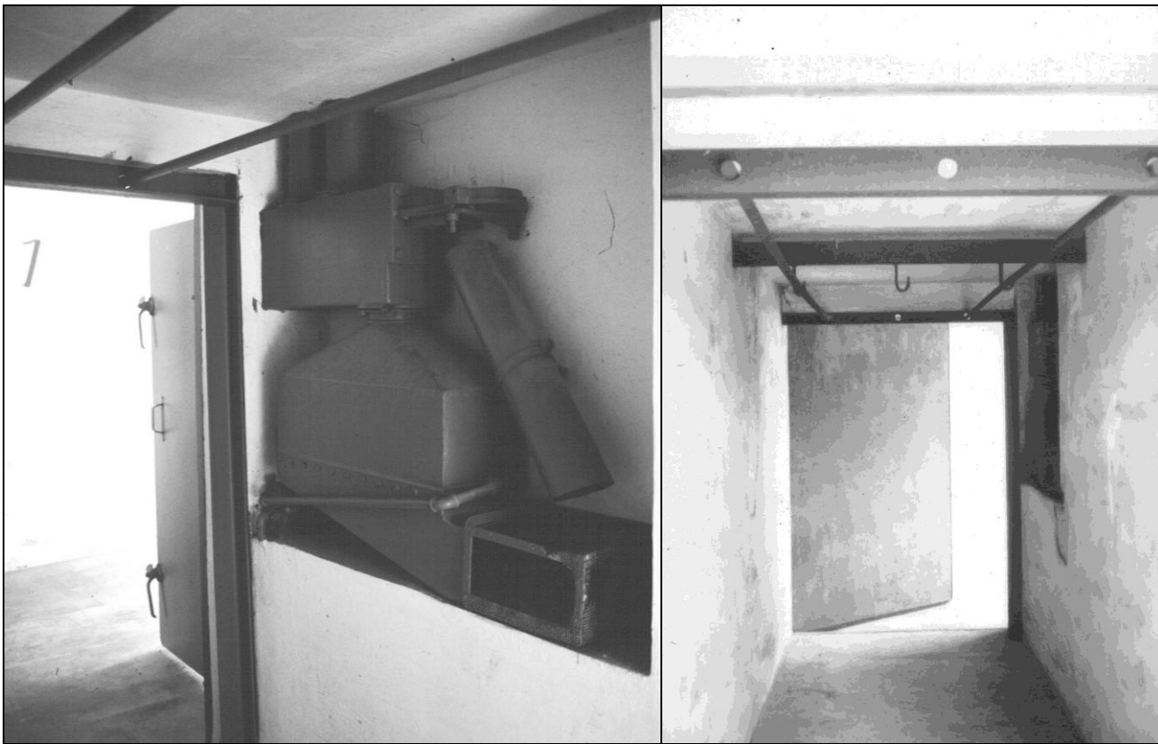
Fig. 6: Interior of disinfestation chamber at Dachau; left: DEGESCH Kreislaufanlage (circulation device); right: look through the chamber. (This photo was taken by the author in 1973.)
